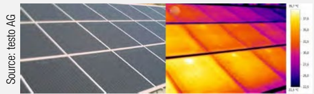
Junction Box Thermogram
