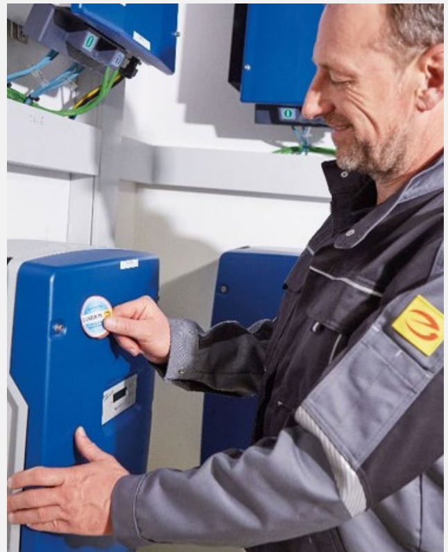
System Inspected – Affix Inspection Seal
